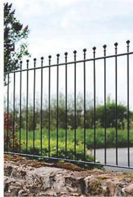
STEEL RAILINGS FIXED TO TOP OF EXISTING WALL AT BACK OF FOOTPATH
